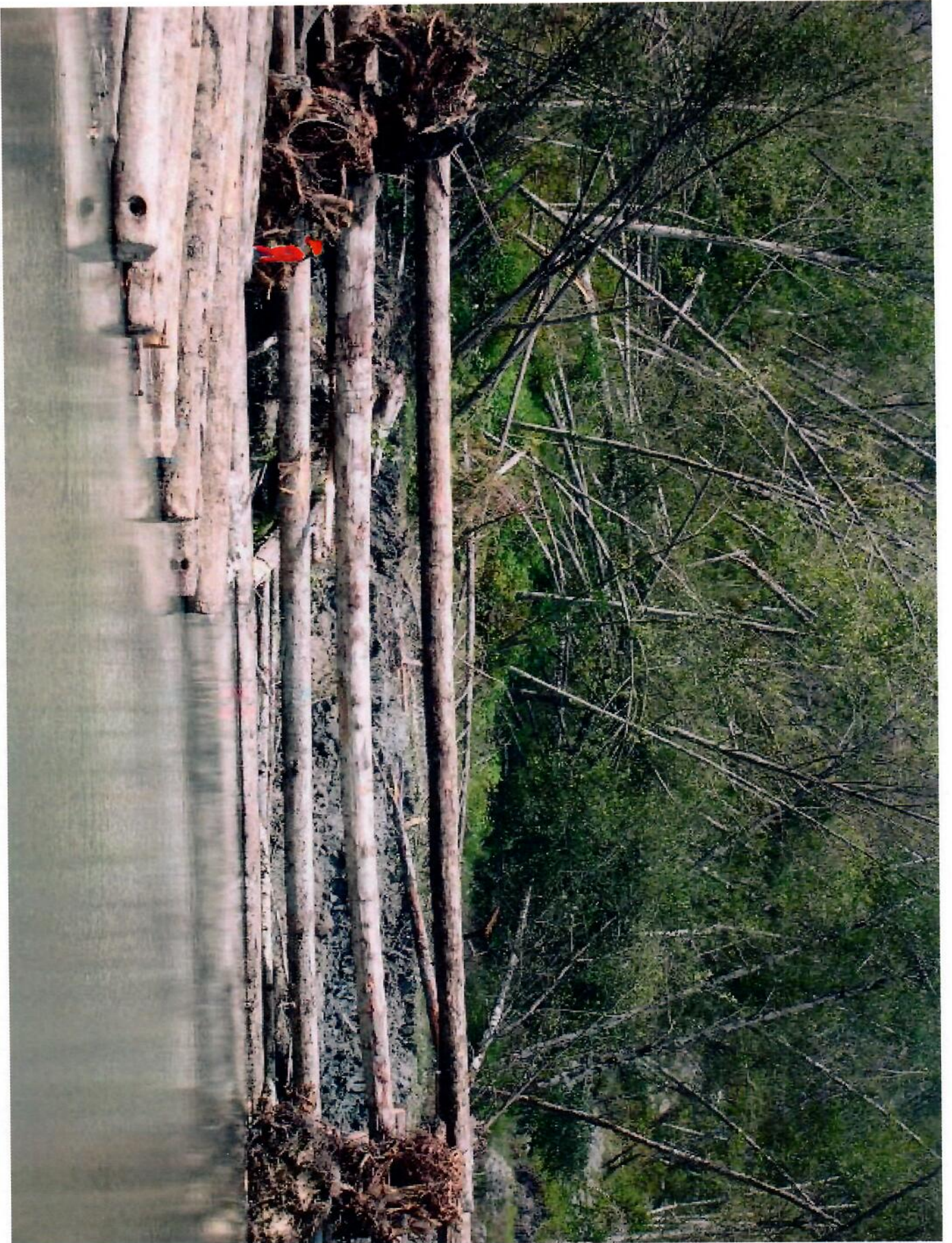
Close up look at log jam revetment. Notice person on left for scale. SC_PDR_WARCO_000159
